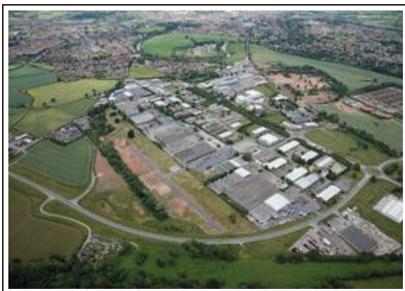
Figure 1.3 – Hereford Enterprise Zone at Rotherwas, Hereford
